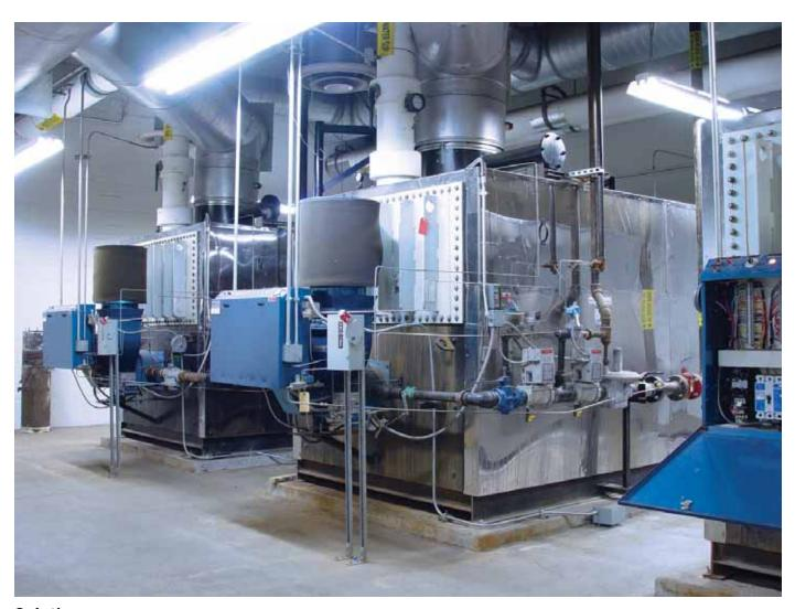
**Solution.** Ajax Boiler supplied three Ajax Series WFG-11500 boilers (11.5 MMBTU/hr per unit). The facility manager uses the three boilers in a lead/lag configuration which gives the convention center the ability to turn boilers on and off to meet varying heat load requirements. Additional benefits include a substantial savings on gas expenses and the ability to shut down a single boiler for service without any interruption in heat for convention center attendees.
